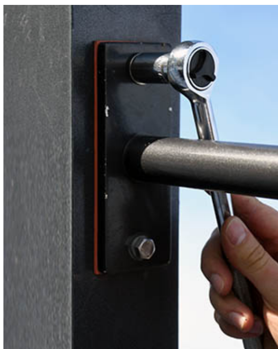
FIGURE 4-10 Weather Arm Bolted to the Pole
