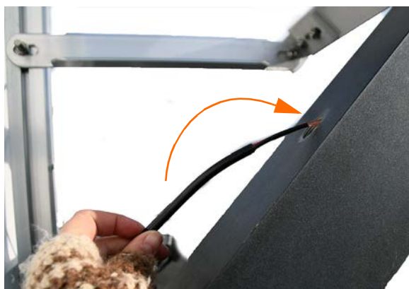
FIGURE 4-2 Feed Cable Down Pole
