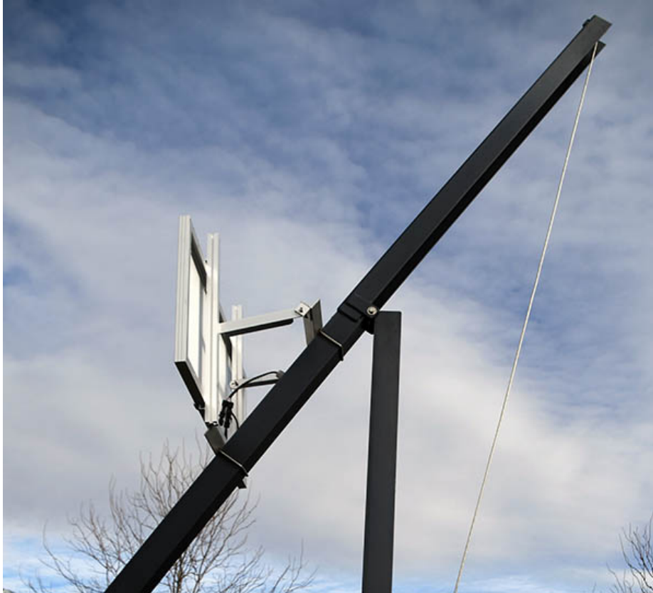
FIGURE 4-7 Solar Panel on Tip-Down Pole
