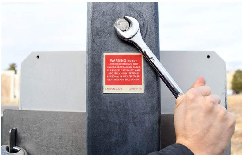
FIGURE 3-2 Remove Bolt from Pole
